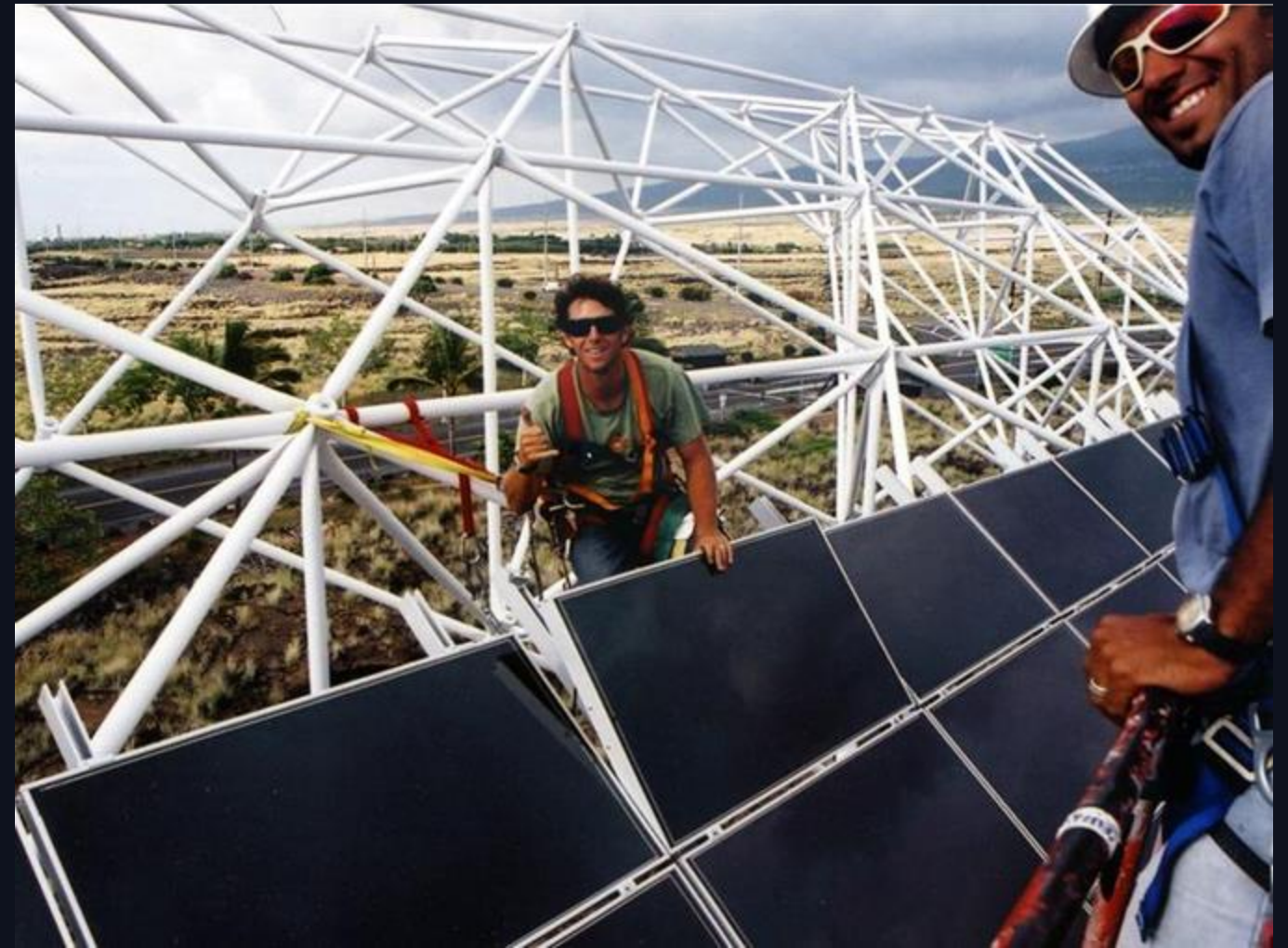
Natural Energy Laboratory Of Hawaii Authority (NELHA) Kona, HI 2003
